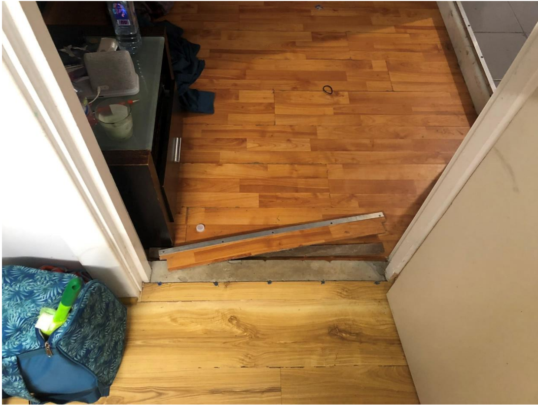
Photograph 4 – Internal floor finishes over concrete slab
